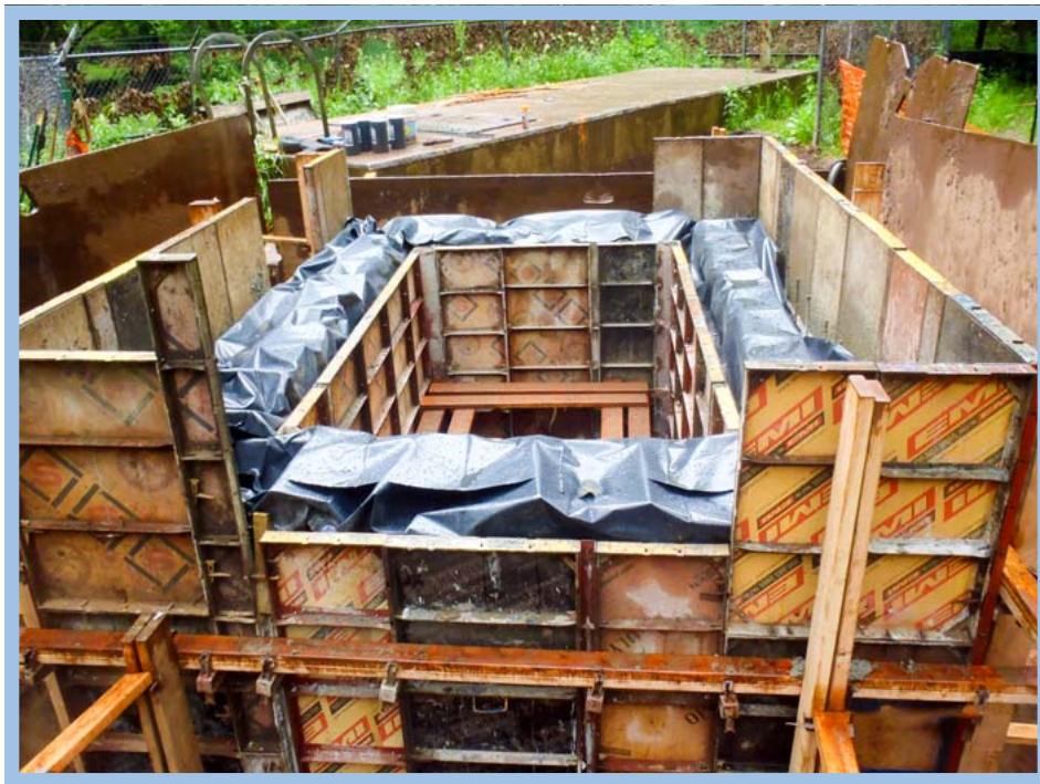
Rehabilitation of the Main Trunk Sewer line.
