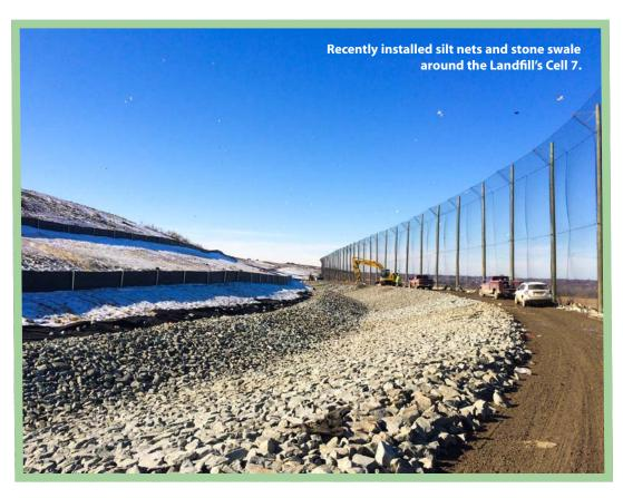
mental Protection Agency, silt netting "ponds sediment-laden stormwater runoff, causing sediment to be retained by the settling processes. A single 100 foot run of silt fence may hold 50 tons of sediment in place."
