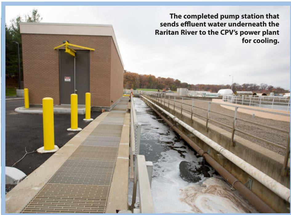
The completed pump station that sends effluent water underneath the Raritan River to the CPV's power plant for cooling.
