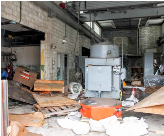
Damage to the Sayreville and Edison Pump Stations following Hurricane Sandy.
