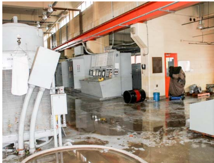
Damage to the Sayreville and Edison Pump Stations following Hurricane Sandy.
