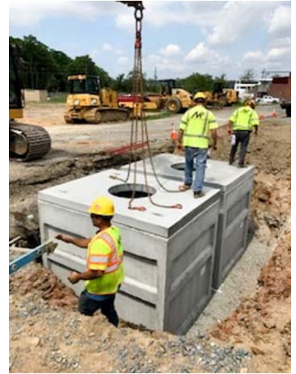
Construction at the Sayreville Pump Station. Above: Manholes in place.
