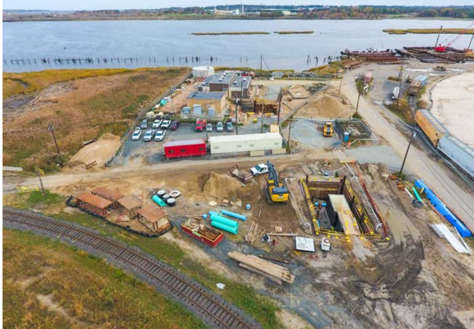
Repairs at the Edison Pump Station.
