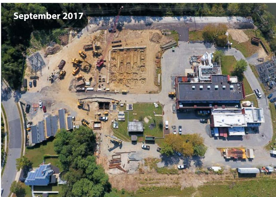
Repairs at the Sayreville Pump Station have been underway for several months. The project includes improvements to the electrical systems and the construction of a perimeter flood wall that will be approximately 1,700 feet long and constructed with a designed top elevation of 21 feet above sea level.
