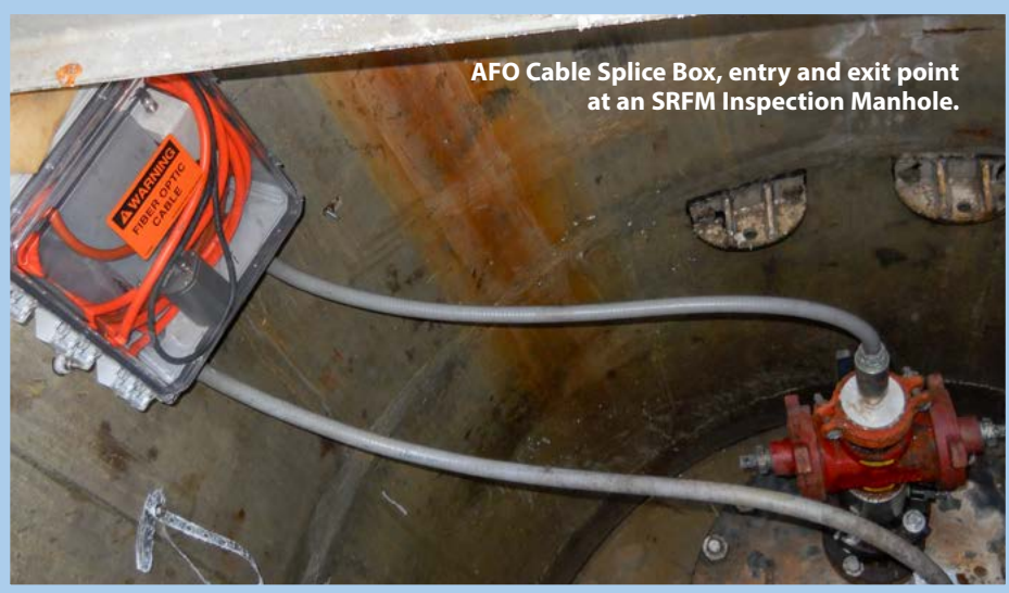
Left: AFO Cable entry and exit point attachment to the inside of the SRFM.
